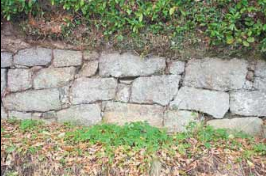
Fig 25 : Granite block wall retaining the churchyard
