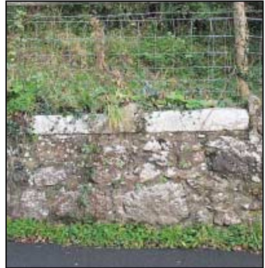
Fig 28: Rubble wall with granite slab coping near Doone Cottage
