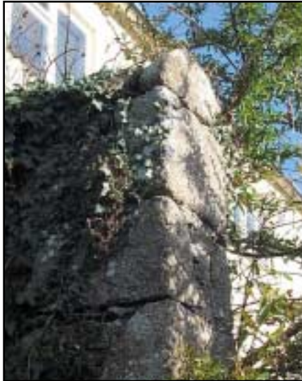
Fig 27: Dressed granite wall at Old School Cottage
