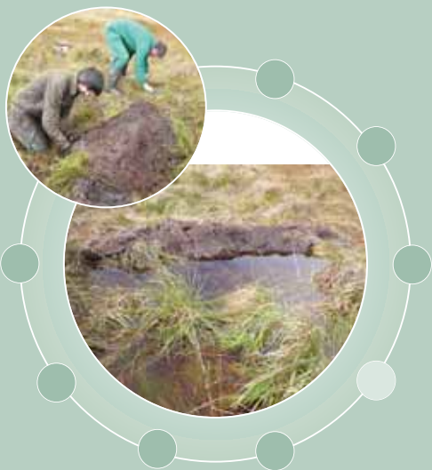
Ditch blocking on blanket bog, Amicombe Hill © AFW
